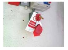
6. A tag should also be used to identify when and who locked out the socket.
