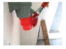
4. Use a HASP to clamp around the socket and the socket lid hinge and through the device fixing position.
