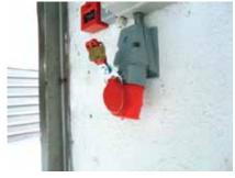
5. Lock HASP in position so it cannot be removed without authorisation. Check device cannot be removed.
